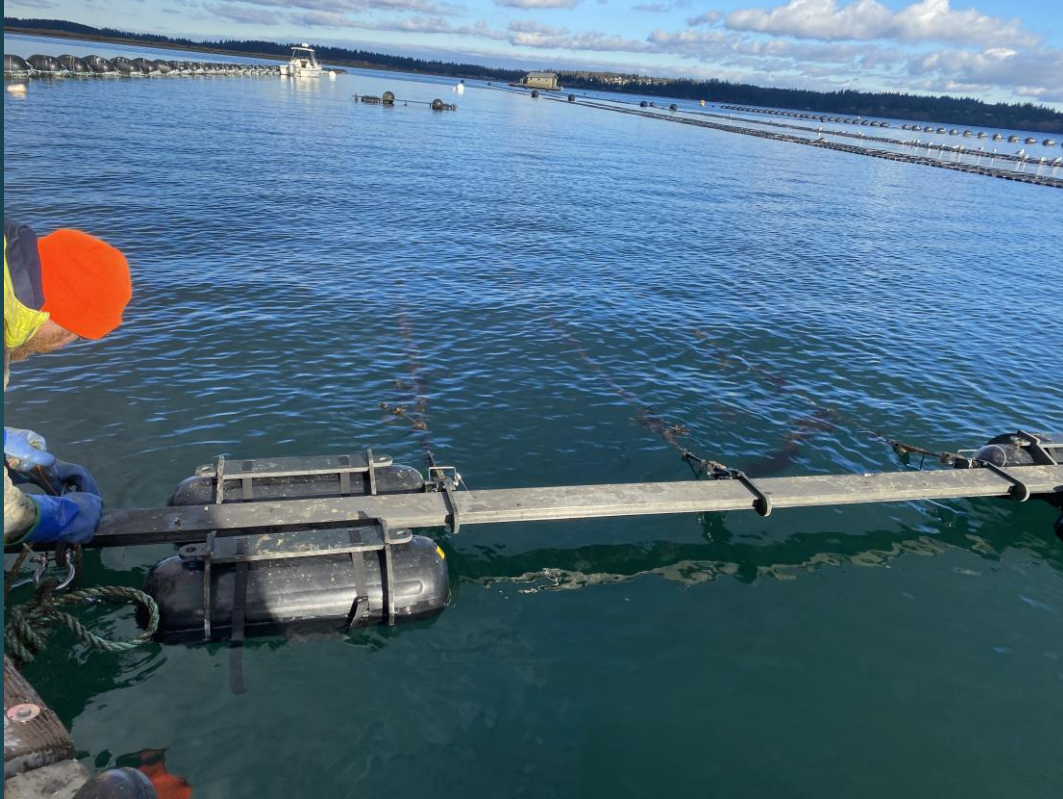
Securing spreader bars on service rafts
