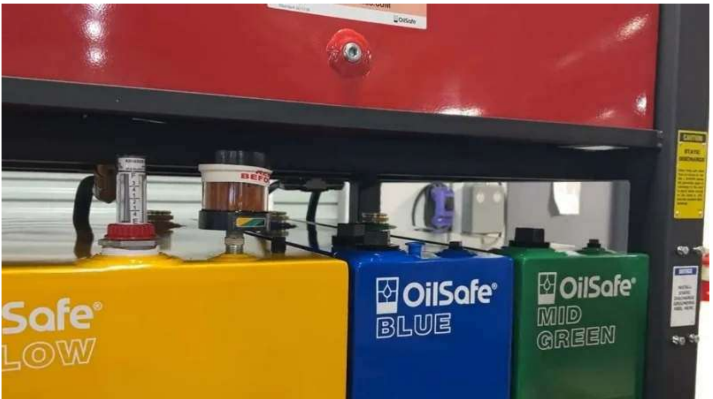
Installing the desiccant breather and adapter
