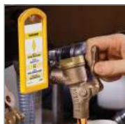
Frame houses labels on Bulk Systems
