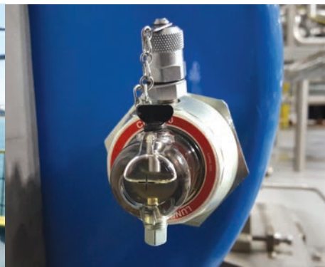
Screw Pump - Bottling Plant
