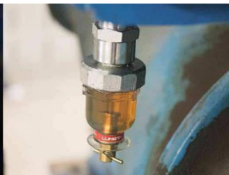
Large Blower - Wastewater Treatment Plant
