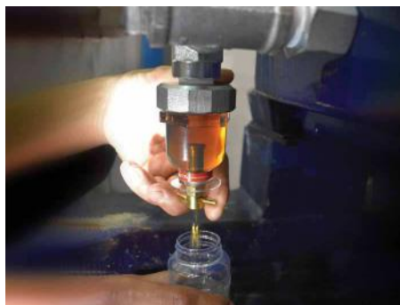
Sludge Pump - Using Bowl to Purge Water and Sediment
