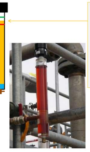
Oil Sight Glass & Level Monitor shows an accurate level of oil inside the reservoir.
