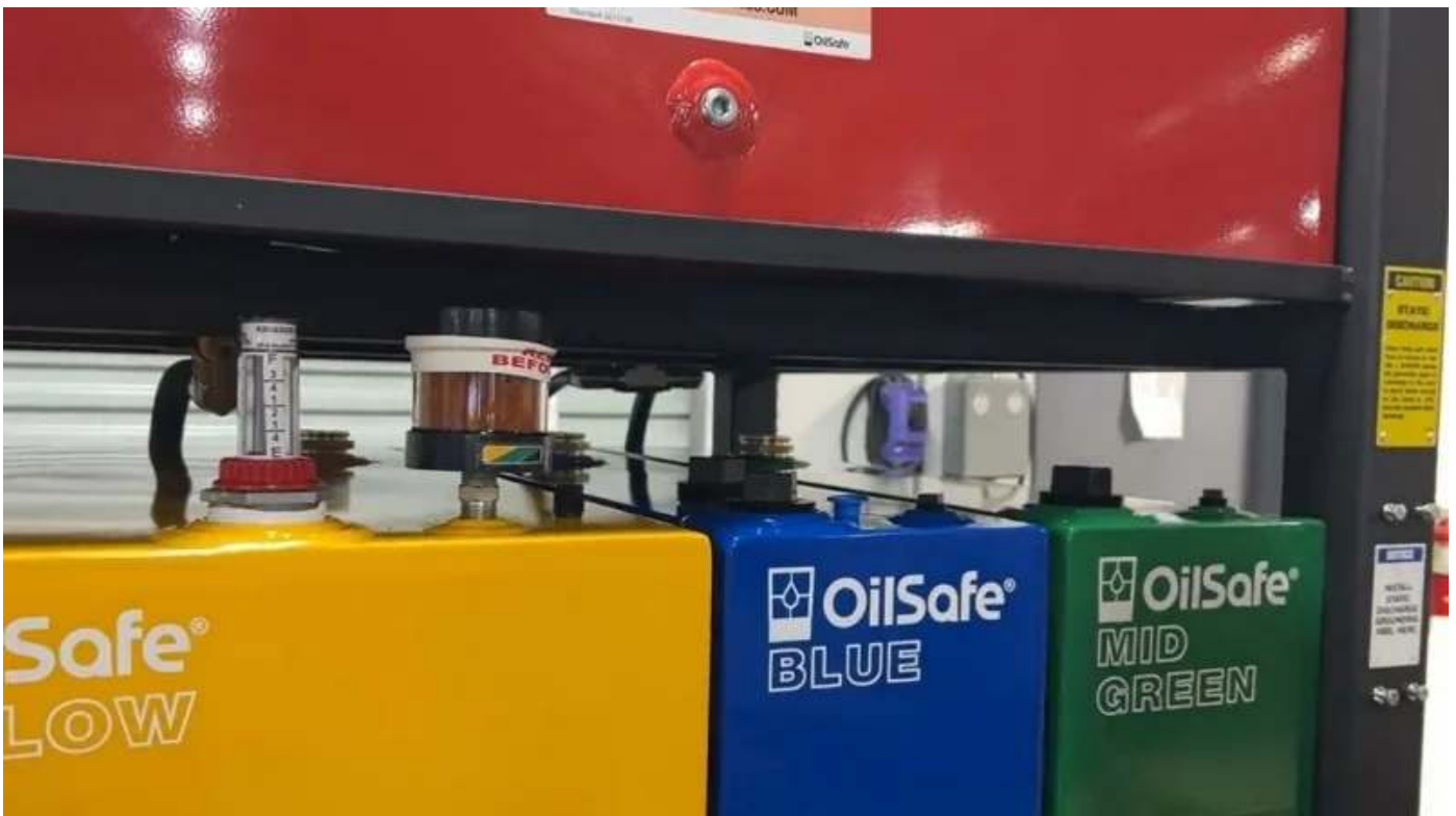
Installing the desiccant breather and adapter
